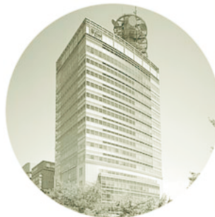
Aluminum structural materials are used in the NTT DoCoMo Nagano Building
