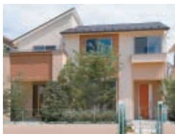
Residential gate and fence
