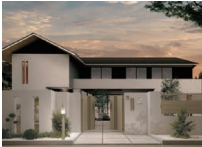
Residential gate and fence
